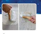
Mix to consistency and apply a first thick coat of MOR-CEMDRY R with a flat brush. Let dry for approximately 2 to 4 hours. Apply a second coat perpendicular to the first one.
