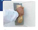
Once the MORCEMDRY R coats have set, apply PEGO-LAND FLEX or PEGOLAND ESPECIAL (depending on degree of absorption of the ceramic tile) by spreading with a notched trowel.
